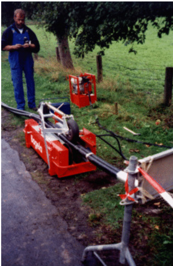
Laying of 3 x single core 30 kV
